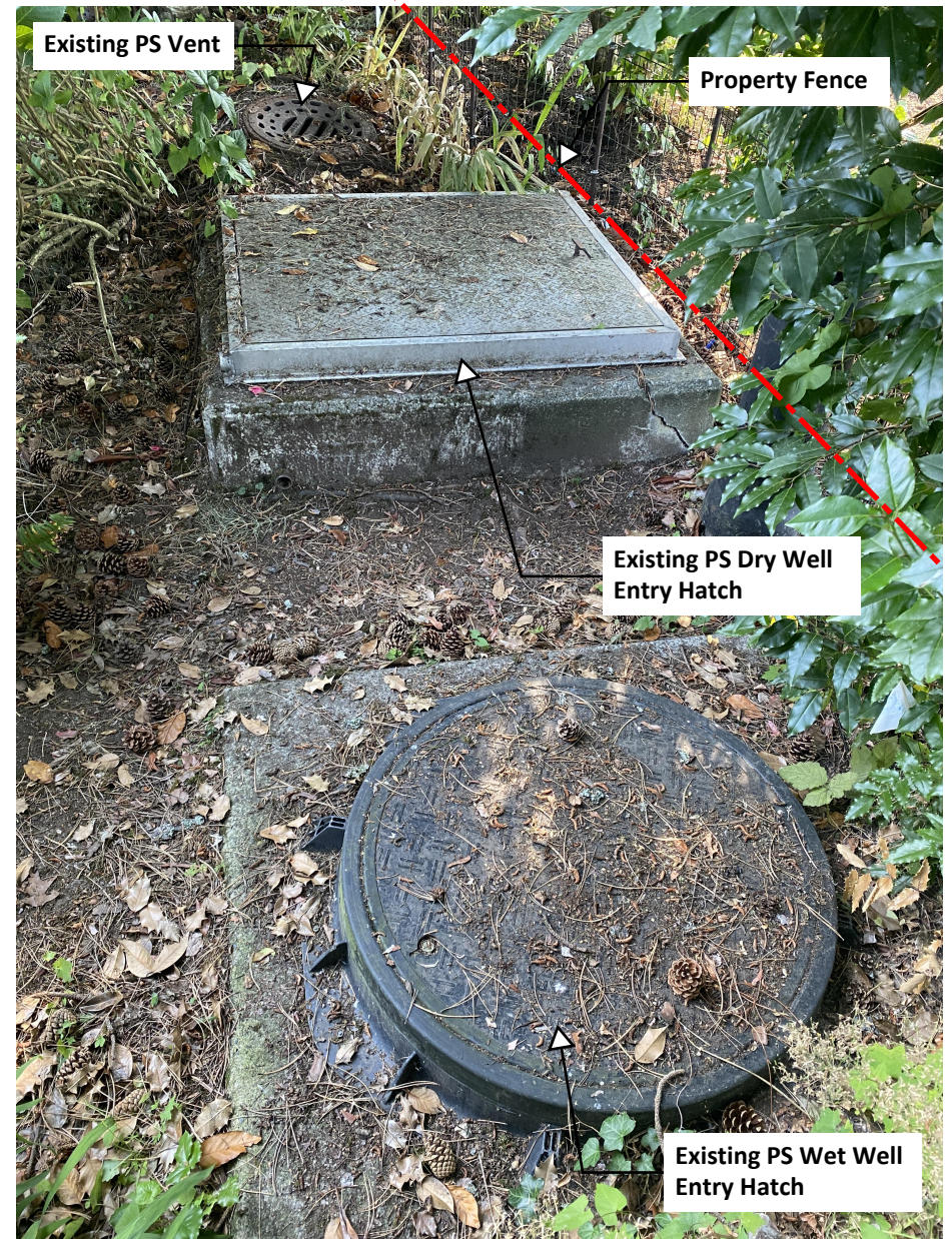
PS17 looking east
